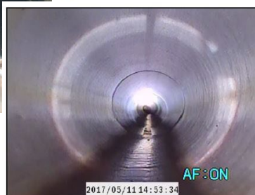
Figure 3-7 Example of a RCP in Excellent Condition (Left) and CMP in Poor Condition (Right)
