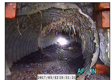
Figure 3-7 Example of a RCP in Excellent Condition (Left) and CMP in Poor Condition (Right)
